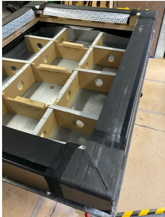
Fig. 3: Elements joined with airtight tape
